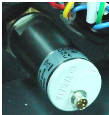
Picture 4-14: Installation for Transmitter
