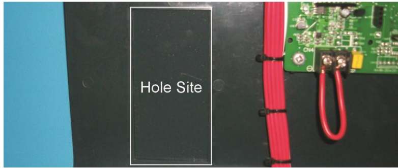
Picture 4-10: Hole Site
