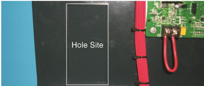
Picture 4-10: Hole Site
