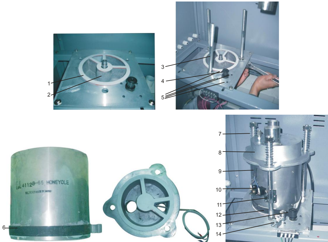
Picture 3-3: Installation of the Rotor
