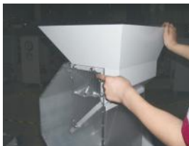
Picture 3-11: Installation of Feed Box, Feed Port and Storage Box 3
