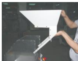
Picture 3-10: Installation of Feed Box, Feed Port and Storage Bin 2
