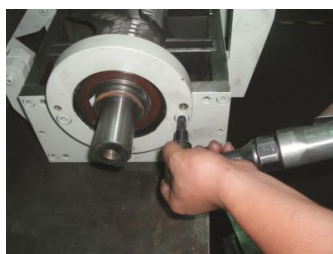
Picture 6-6: Installation of Bearing and Cutter Shaft 3
