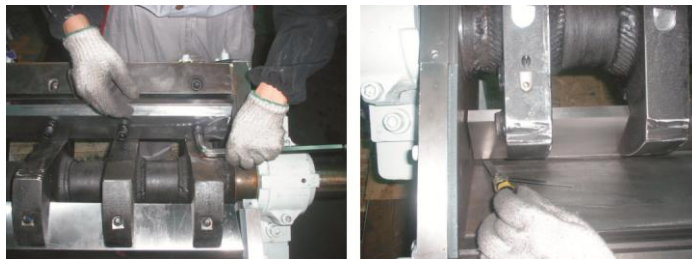
Picture 3-15: Installation of Fixed Blades and Rotating Blades
