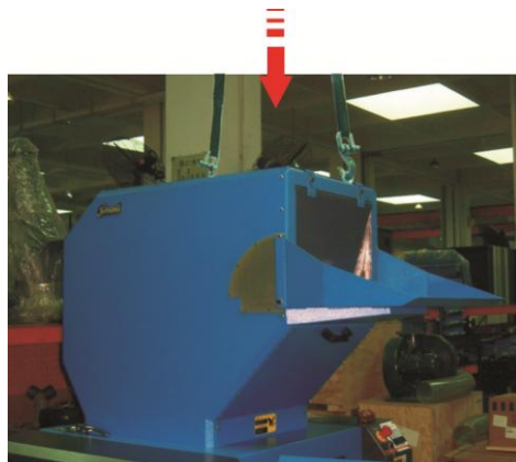
Picture 3-17: Installation of Feed Box and Feed Inletv 1
