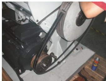
Picture 3-8: Installation of Belt Pulley and Motor 2(SG-3650)
