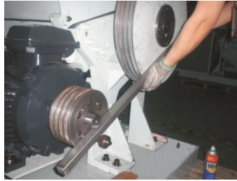
Picture 3-9: Installation of Belt Pulley and Motor 2 (SG-3650)
