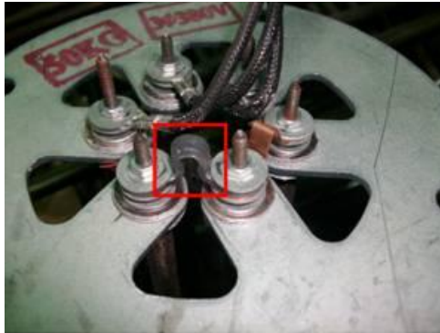
Picture 4-3: Lead sheet fuse
