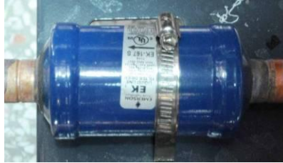
Picture 2-29: Drying Filter
