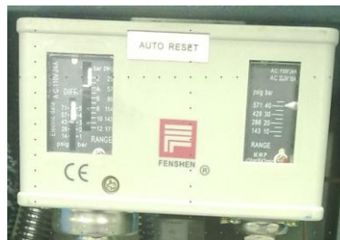
Picture 2-32: High and Low Pressure Controller
