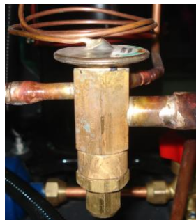
Picture 2-30: Heat Expansion Valve
