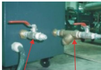
Cooling water outlet Cooling water inlet
